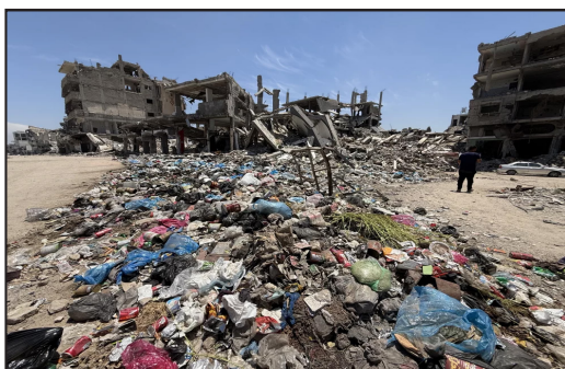
Piles of uncollected garbage and debris line a deserted street in al-Shuja'iyya, a neighborhood lacking basic services and aid due to Israel restrictions as expanding the orange zone.
